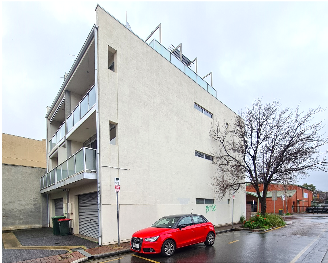
Photo 3.5 – Adjacent dwellings at 122 Gilles Street, Adelaide
